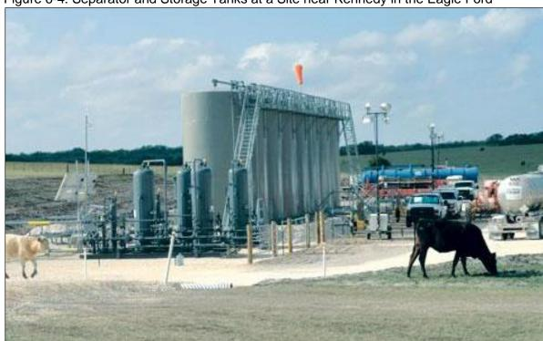
Figure 6-4: Separator and Storage Tanks at a Site near Kennedy in the Eagle Ford
