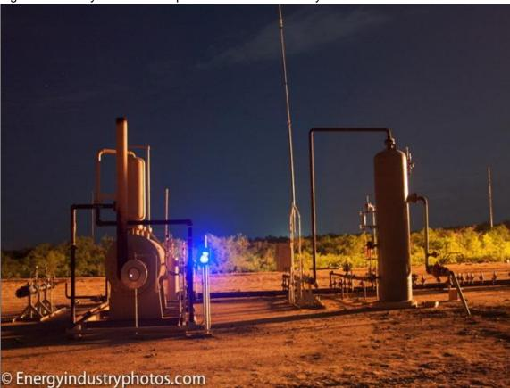
Figure 6-3: Dehydrator and Separator in Karnes County
