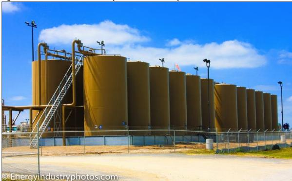
Figure 7-3: Centralized Tank Battery in Gonzales County<sup>355</sup>
