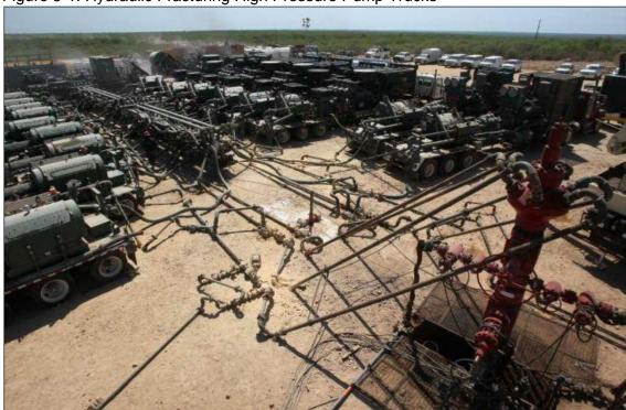
Figure 5-1: Hydraulic Fracturing High Pressure Pump Trucks<sup>198</sup>
